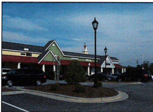
Shopping Center at Lewisville-Clemmons Road/Styers Ferry and HWY 421
