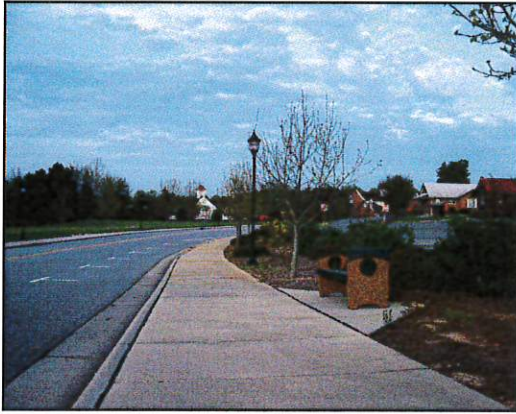
Great Wagon Road Streetscape behind Roller Mill
